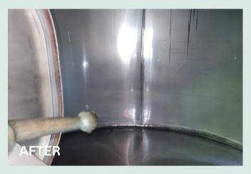
Images showing inside of tanks before and after using 0.6% v/v Circlean Phosphate Free cleaning via a venturi system with 200L of cold water for 20 minutes.
