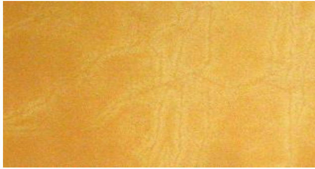
Concrete surface crazing showing colour variation due to moisture & salts
