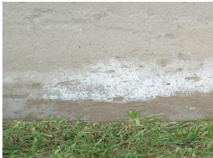
Salts on unsealed concrete adjacent to grass
