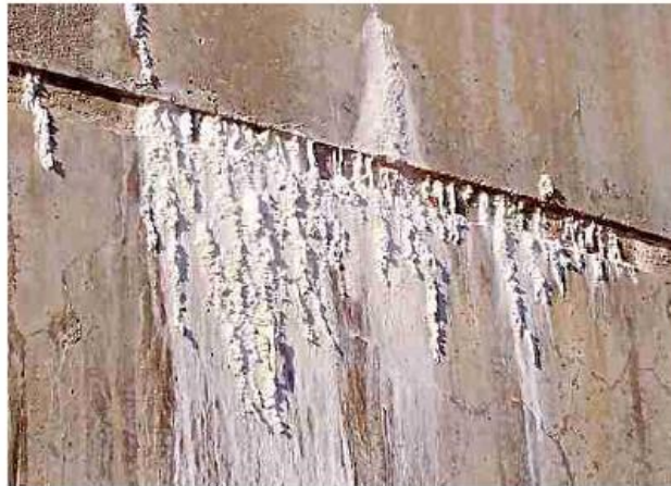
Calcium Carbonate salts
