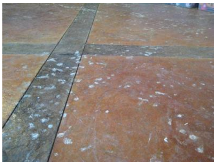
Salts patches on coloured concrete paving
