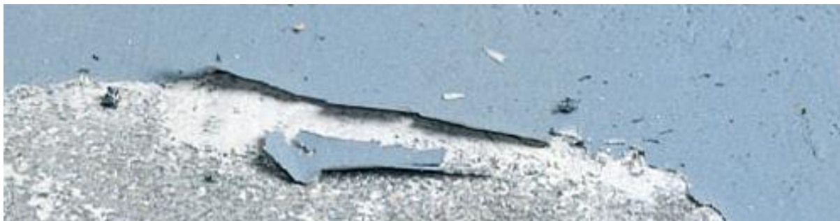
Sealer lifting due to salts underneath. Poor surface penetration and lack of adhesion very apparent due to incorrect application.
