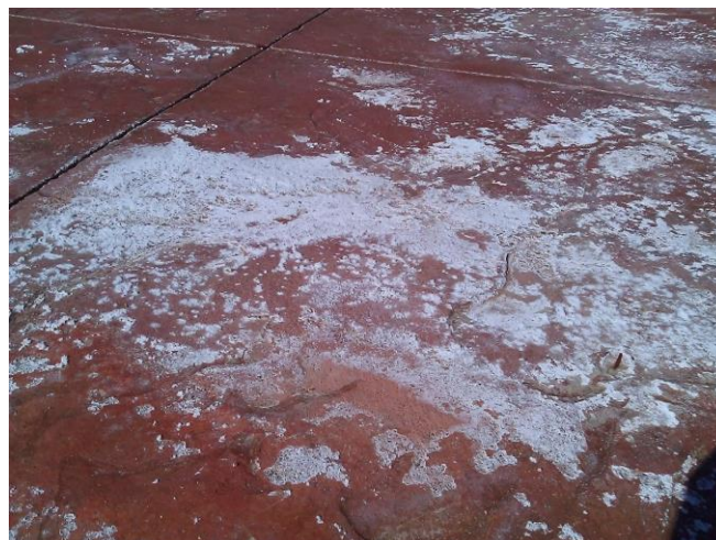
Salts on slate impression concrete where the sealer has delaminated
