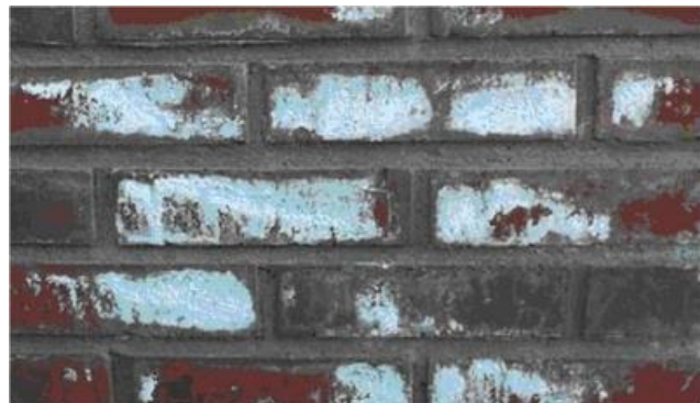
Salts on a brick wall caused by rising damp
